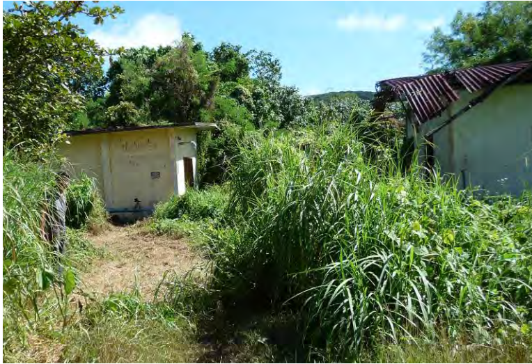
Figure 1: Maui I Well Pump House to the left, operations building to the right
