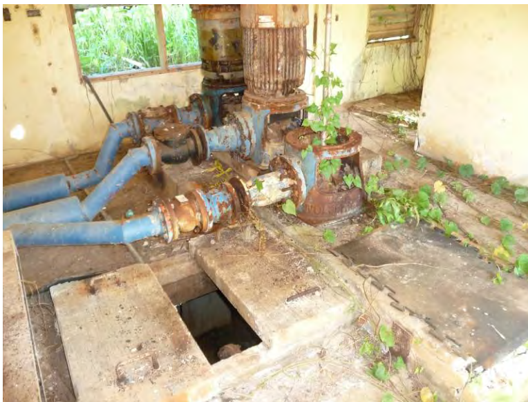
Figure 2: Maui I Pumps
