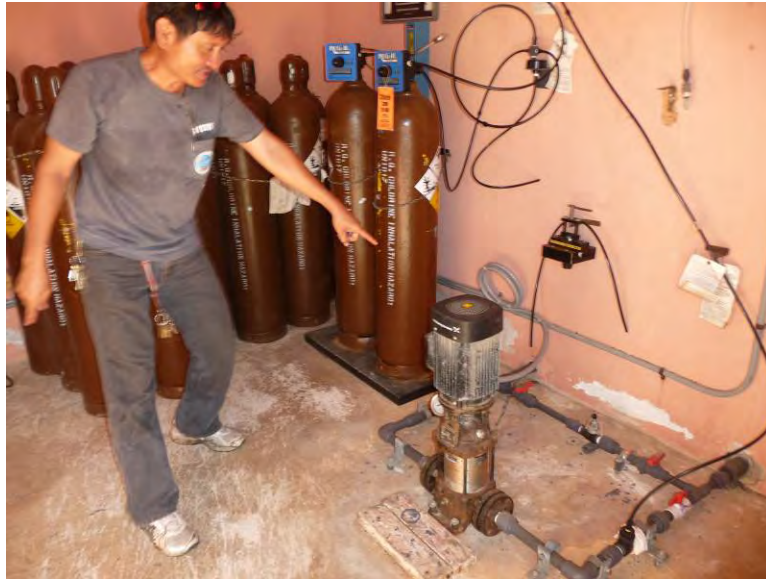
Figure 13: Chlorination system at Maui II Well Facility.
