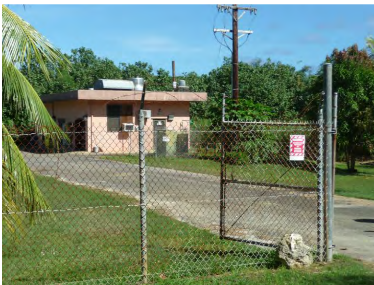
Figure 6: Maui II Well Facility
