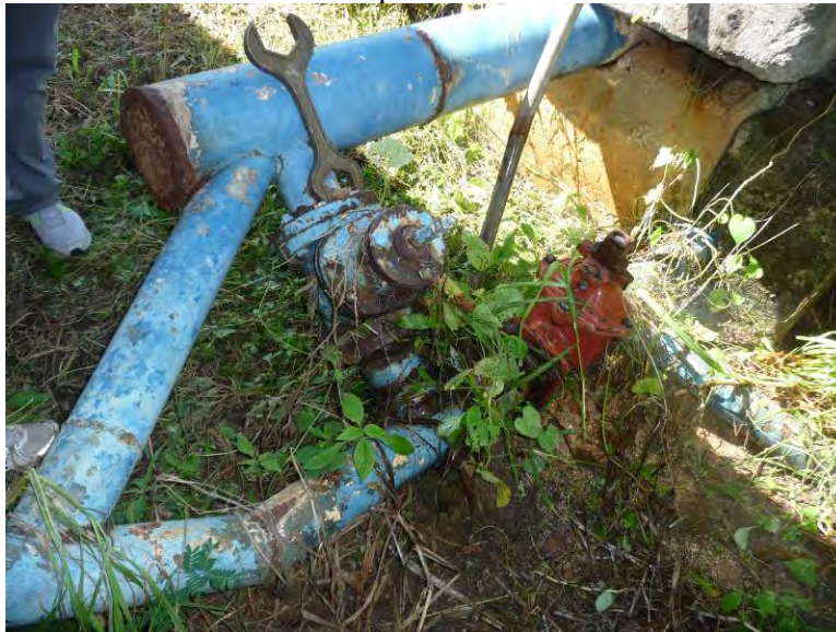
Figure 4: Pipe manifold (discharge side of Maui I Well)
