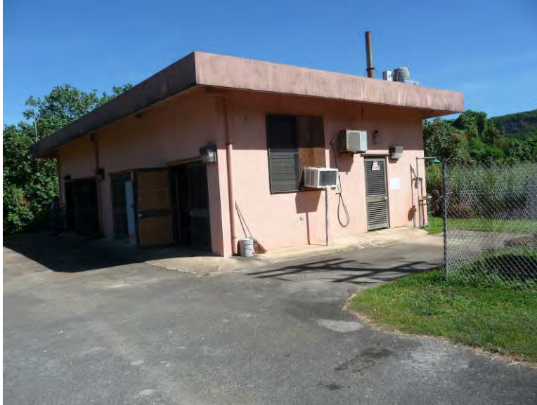
Figure 6: Maui II Well Facility
