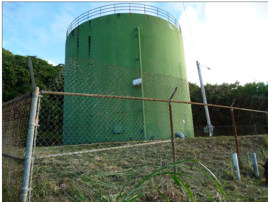
Photo 2.1-7. Carolinas Water Storage Tank (Half Million Gallon Tank)
