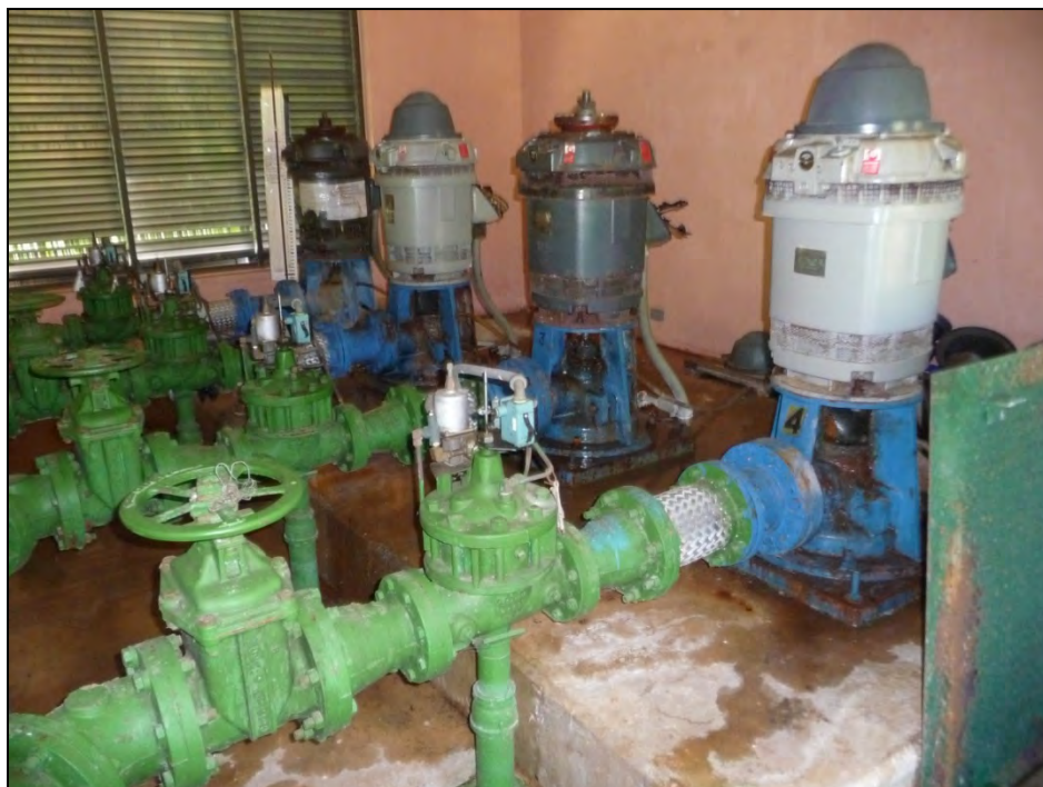
Photo 2.1-4. Maui Well No. 2 Pump Equipment
