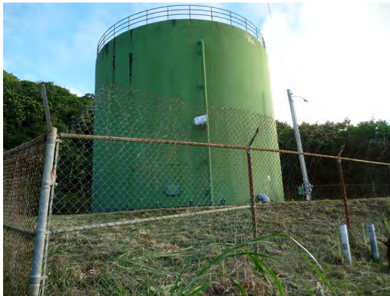
Figure 14: Half Million Gallon Tank (HMT)
