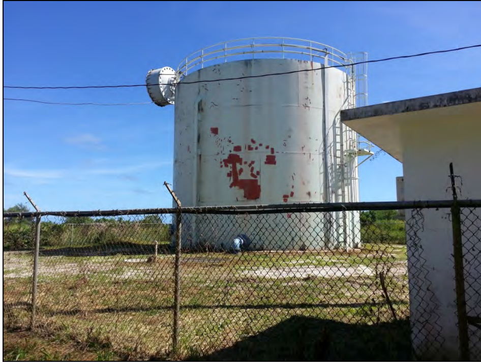
Photo 2.1-6. Marpo Heights Water Storage Tank (Quarter Million Gallon Tank)
