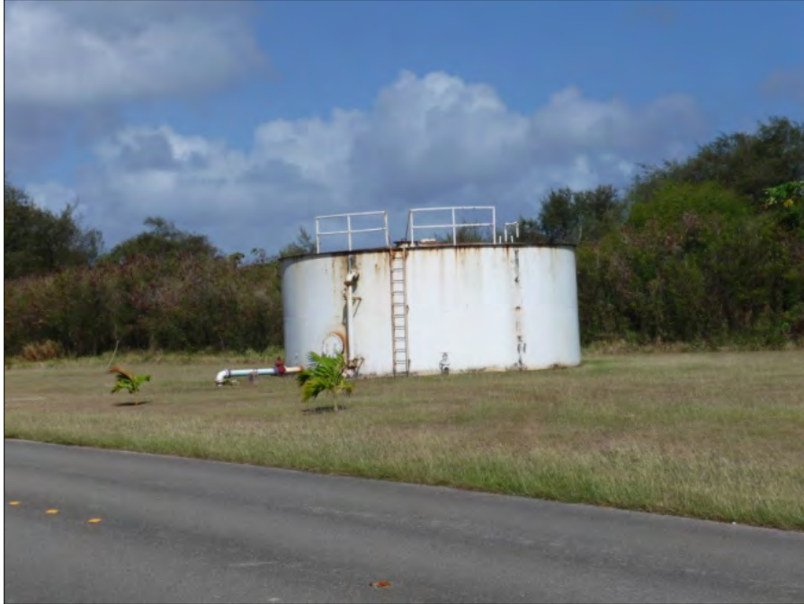
Photo 2.1-8. Tinian Airport Water Storage Tank
