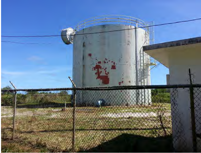
Figure 15: Quarter Million Gallon Tank (QMT)
