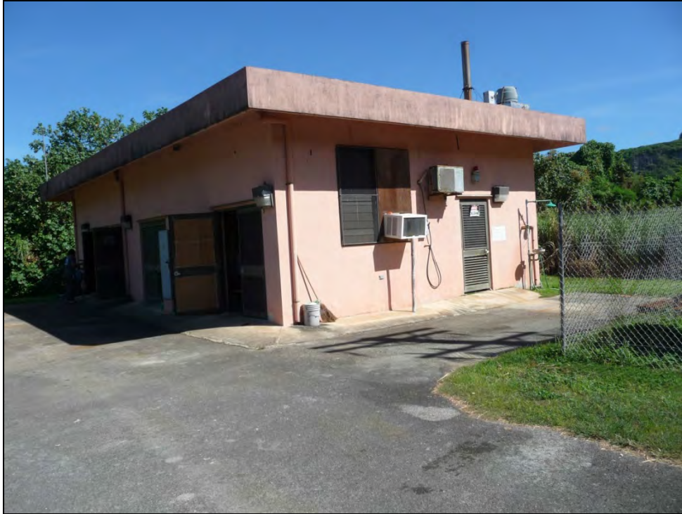
Photo 2.1-3. Maui Well No. 2 Pump House
