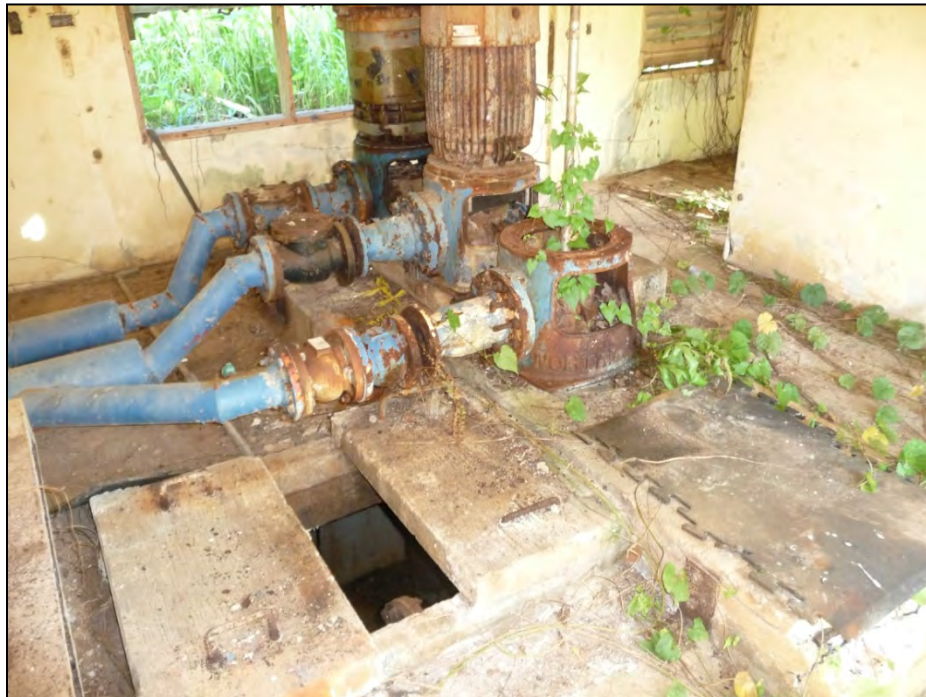
Photo 2.1-2. Maui Well No. 1 Pump Equipment
